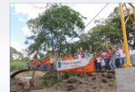
El Limón Bridge, Nicaragua This foot-bridge serves to link locals to schools, medical care, and markets on the other side of the river during the rainy season.
