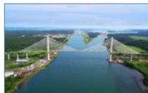
Cable-Stayed Concrete Bridge 3rd PANAMA CANAL CROSSING Colón, Panama Main Span: 530 m (1,738 ft)
