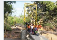
El Corozo Bridge, Nicaragua The footbridge provides safe access to schools, health care, markets, government services, and employment opportunities to four rural communities.
