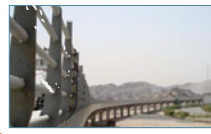
Fast-Track Metro Design MASHAAER MMMP MECCA, Saudi Arabia Design and Construction Supervision in 17 mos. Total Length: 17 km (10.6 mi)
