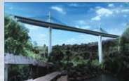
Mauritius Extradosed Bridge, Mauritius Island SYSTRA proposed an alternate concept design with savings of 39% in concrete, 33% in reinforcing steel and 20% in stay cables, compared with the existing design.
