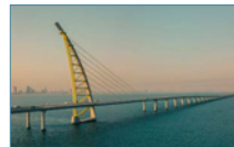
Sea Bridge SHEIKH JABER AL-AHMAD AL-SABAH CAUSEWAY, Kuwait Total Length: 48.5 km (30.1 mi)
