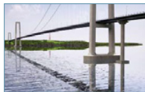
Suspension Bridge CHACAO BRIDGE, Chacao, Chile Main Spans: 1,155 m (3,789 ft) and 1,055 m (3,461 ft)
