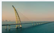
Sheikh Jaber Al-Ahmad Al-Sabah Causeway, Kuwait 140 thousand CO2 tons compared to base design.
