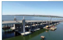
Floating Bridge EVERGREEN POINT FLOATING BRIDGE Seattle, Washington Total Bridge Length: 5,135 ft (1,565 m)
