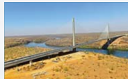
Chambal Bridge, India Noise barriers were installed on the deck to avoid disturbing river crocodiles.
