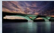
Kingston Third Crossing, Canada Placing an environmental turbidity curtain and wildlife passages, allowing safe passage of turtles and wildlife through the temporary rock causeway during construction.
